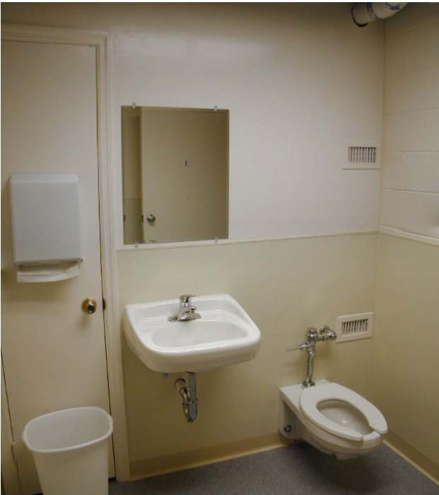
Pictures of the Basement Bathroom Project (preceding page.) and completed bathroom above.
